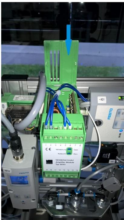
4. Set the DIP-switch as shown in the circuit diagram
